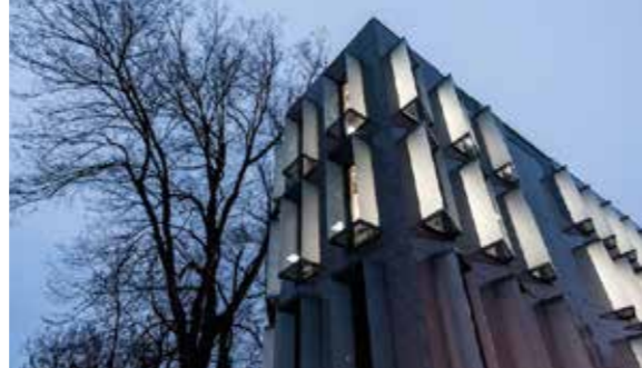
PLATOU CLARKSON OFFICES BUILDING - OSLO (NORWAY)
