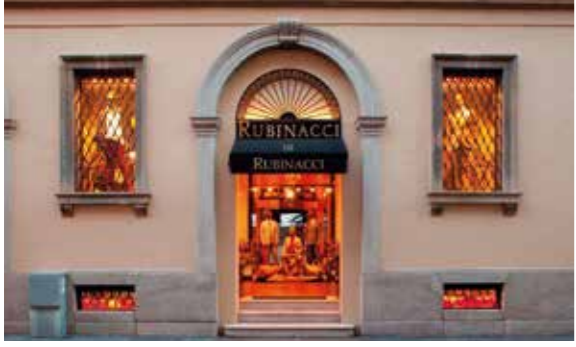
ATELIER RUBINACCI BUILDING - MILANO (ITALY)
